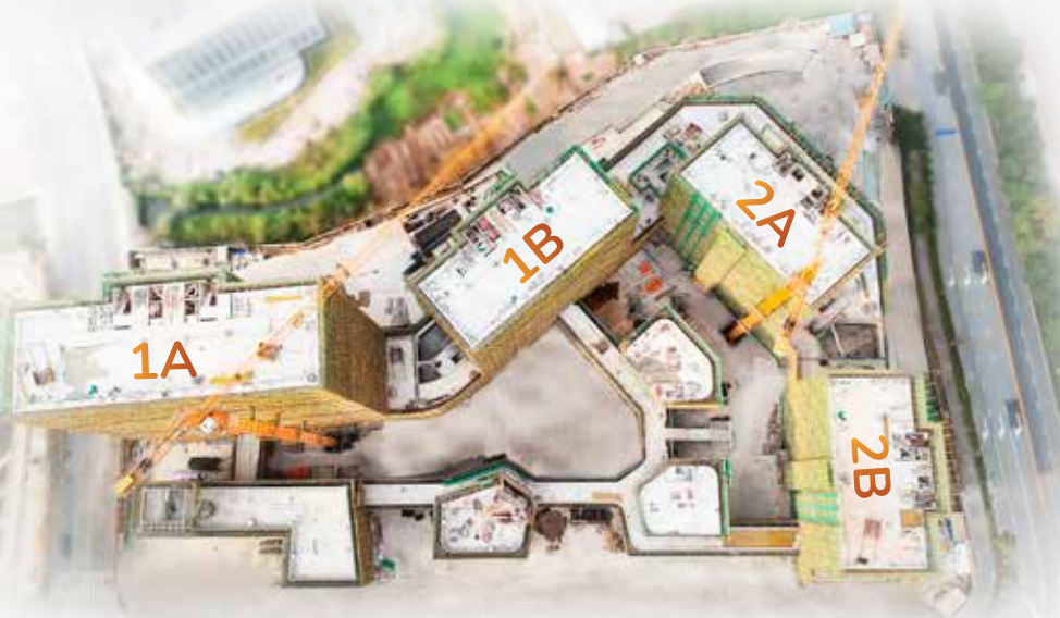
APEX TOWER (AS AT 23 JAN 2020)
